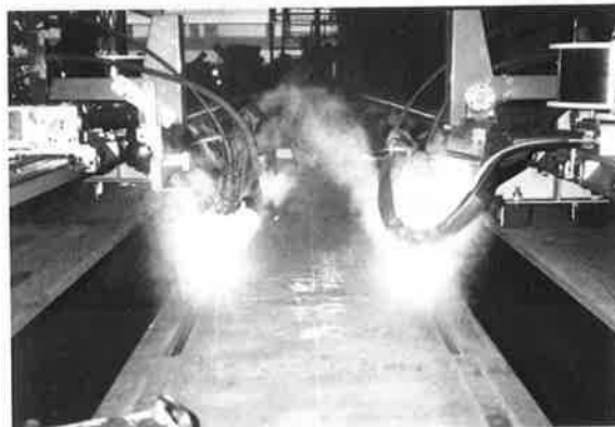
(c) 溶接状況
