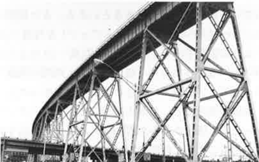
写真-16 HUEY P. LONG BRIDGE
