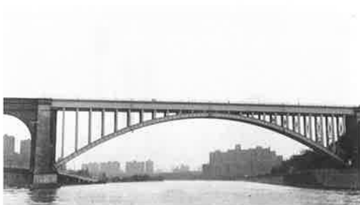
写真-38 HIGH BRIDGE ( ⑱ )
