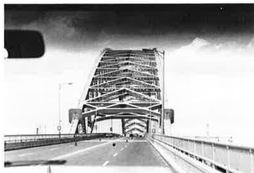
写真-46 BAYONNE BRIDGE ( 27 )
