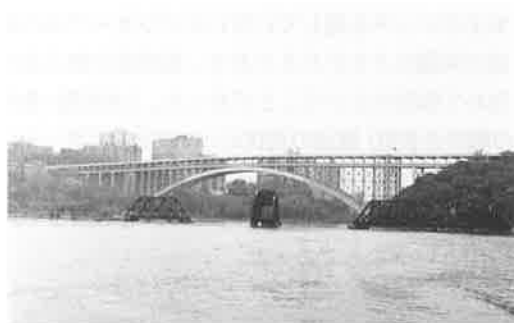
写真-42 (アーチ橋) HENRRY HUDSON BRIDGE ( ㉓ ) (トラス橋) SPUYTEN DUYUIL BRIDGE ( ㉔ )
