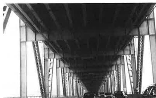
写真-3 RICHMOND SAN RAFAEL BRIDGE
