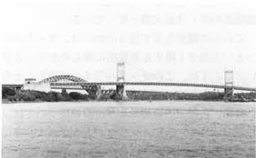
写真-29 (吊橋) TRIBOROUGH (EAST) BRIDGE ( ⑤ ) (アーチ橋) HELL GATE BRIDGE ( ⑥ )
