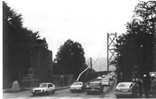
写真-49 LIONS GATE BRIDGE
