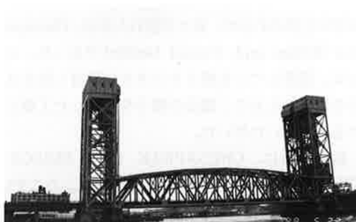
写真-34 PAN-CENTRAL RR BRIDGE ( ⑭ )
