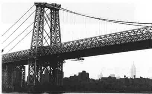
写真-27 WILLIAMSBURG BRIDGE ( ③ )
