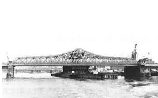
写真-33 3rd. AVENUE BRIDGE ( ⑬ )
