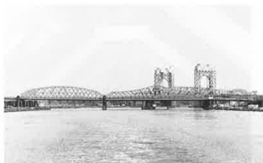
写真-32 WILLIS AVENUE BRIDGE ( ⑫ )
