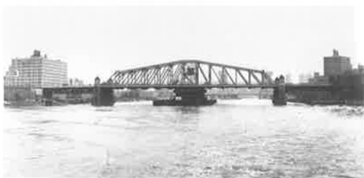
写真-36 14th. STREET BRIDGE ( ⑯ )
