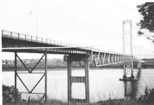
写真-54 TACOMA NARROWS BRIDGE
