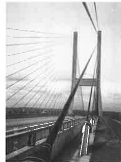
写真-51 ANNACIS BRIDGE
