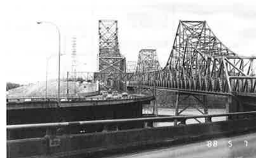
写真-4 CARQUINEZ BRIDGE
