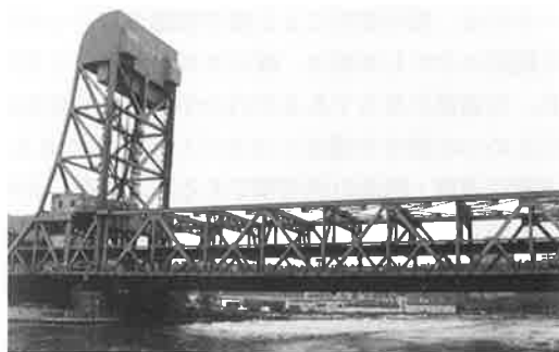
写真-41 225th. STREET BRIDGE ( ㉒ )
