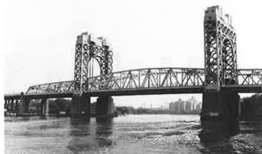
写真-31 TRIBOROUGH (HARLEM) BRIDGE ( ⑩ )
