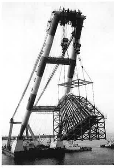
写真-4 吊り曳航
