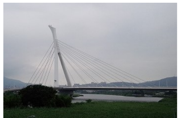
写真-8 Shezi Bridge
